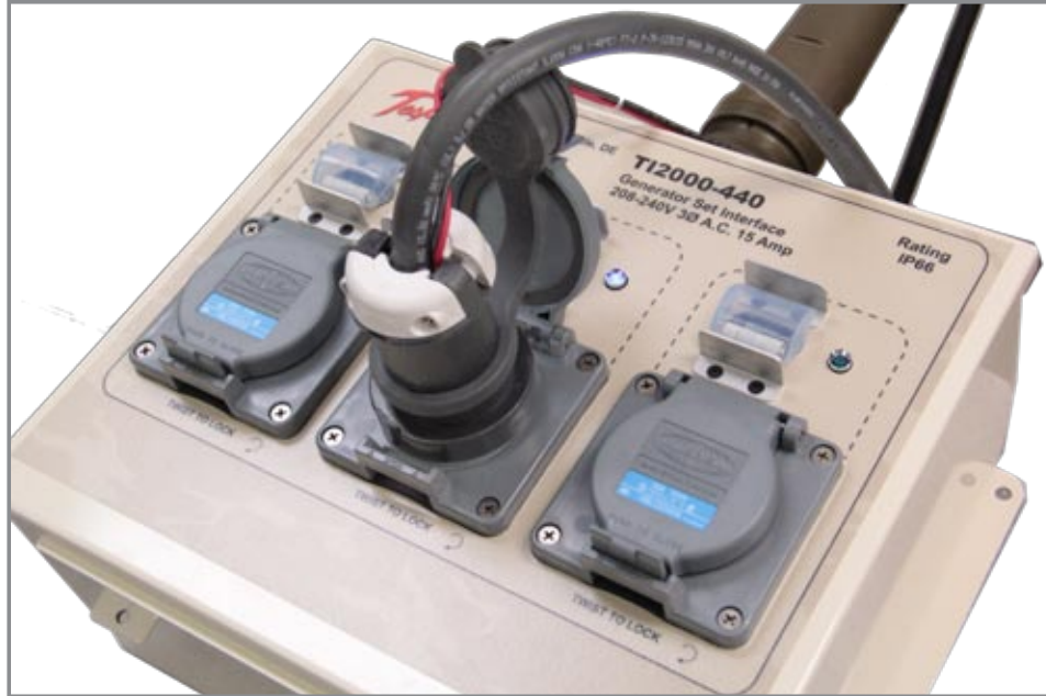
Figure 3.4.6 TI3000 GPU-24 plugged into TI2000-440 with circuit breaker turned on.
